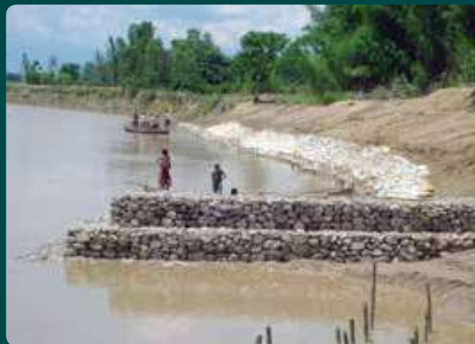
Figure 42: Gabion spurs with sandbags along the bank
