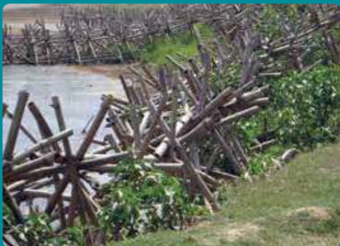
Figure 63: Bamboo porcupines as protection along an embankment
