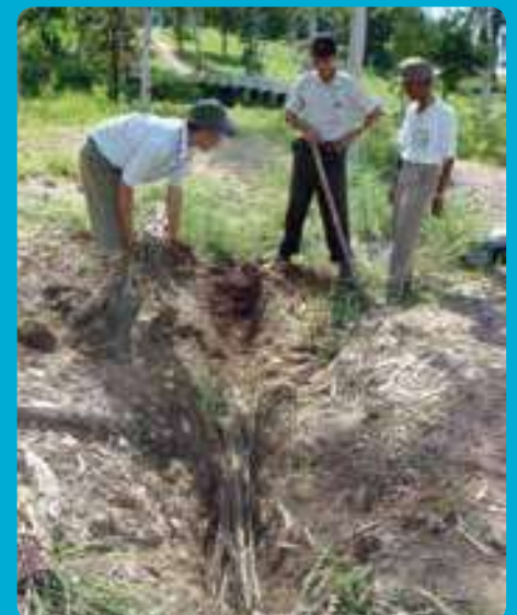
Figure 18: Installing live fascine
