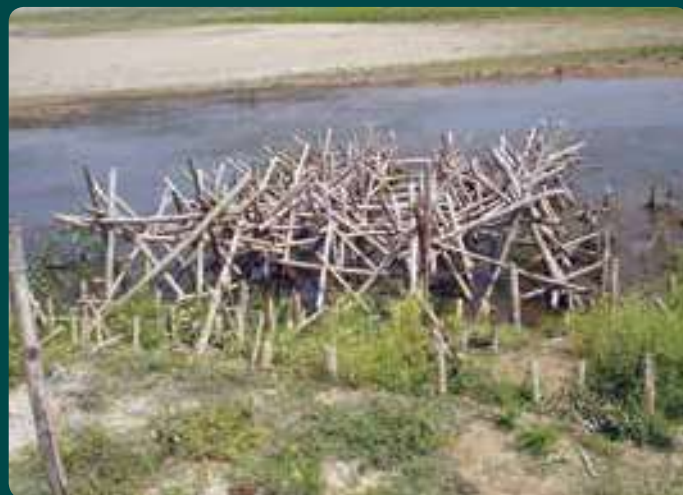
Figure 50: Bamboo porcupines used to form a spur
