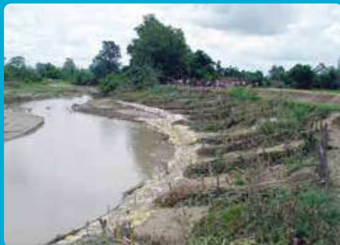
Figure 44: Low-cost spurs made from tree trunks and branches
