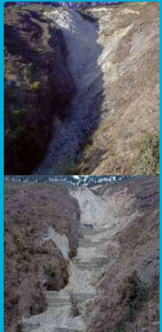
Figure 36: Gully erosion (top) and check dam treatment (bottom) in Dahachowk, Kathmandu, Nepal
