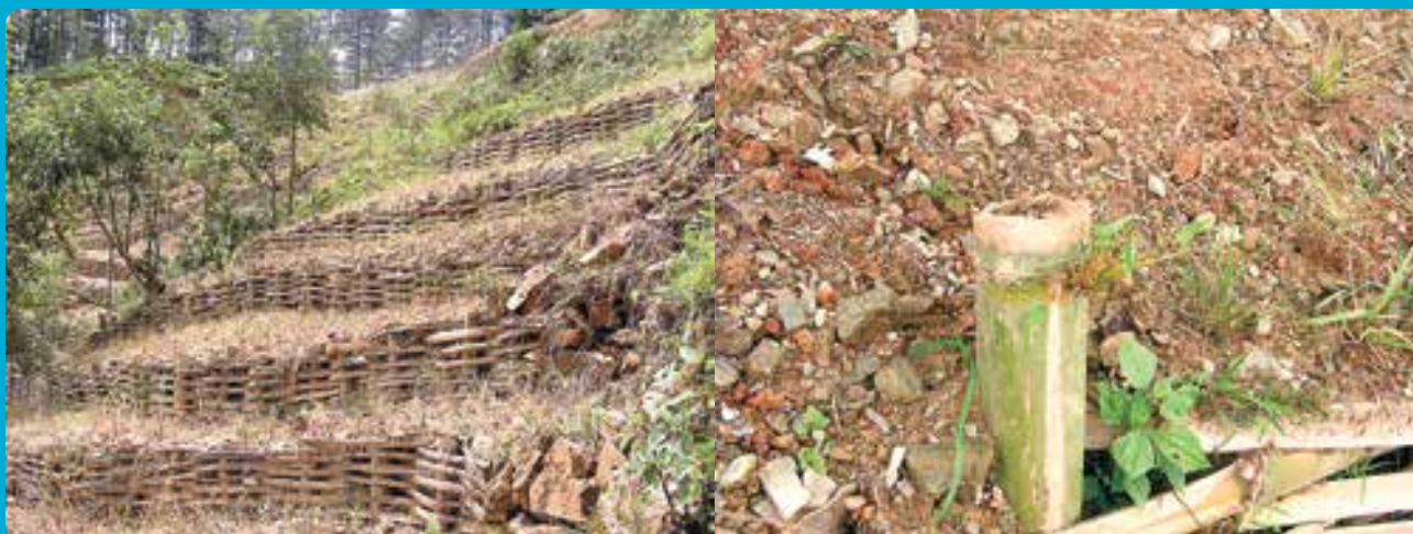
Figure 8: Bamboo fencing on a slope – the posts (pegs) are live bamboo that will sprout to provide foliage (left); detail showing live bamboo peg with sprouting leaves (right)
