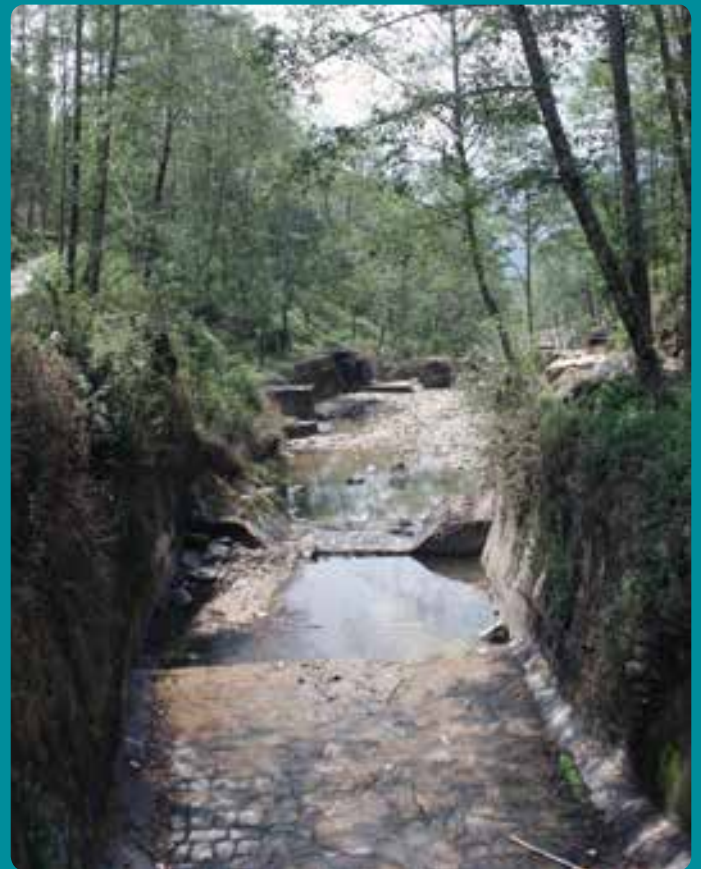
Figure 67: Concrete channel lining
