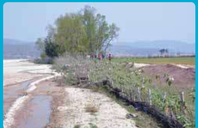
Figure 21: Wattle fence used for river bank protection
