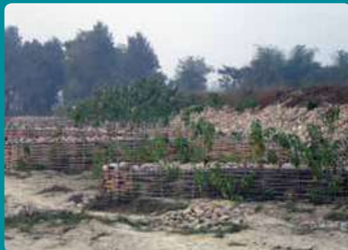
Figure 43: Low-cost bamboo and stone spurs
