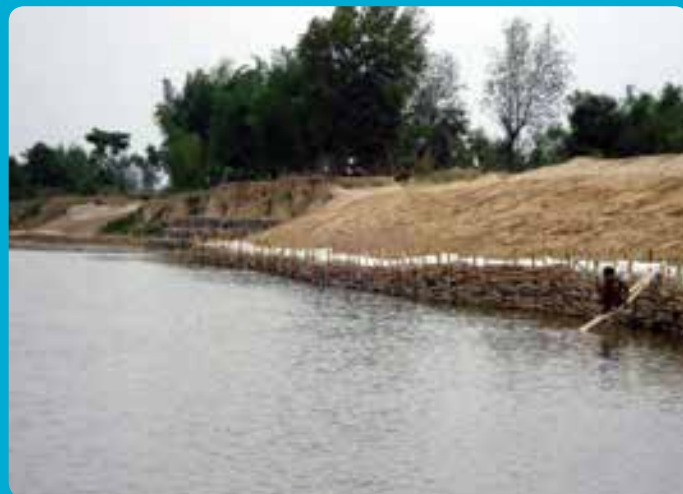
Figure 64: Toe wall constructed from bamboo and sandbags
