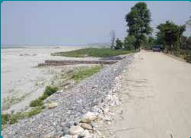
Figure 55: Levee along the Rapti River in Nepal
