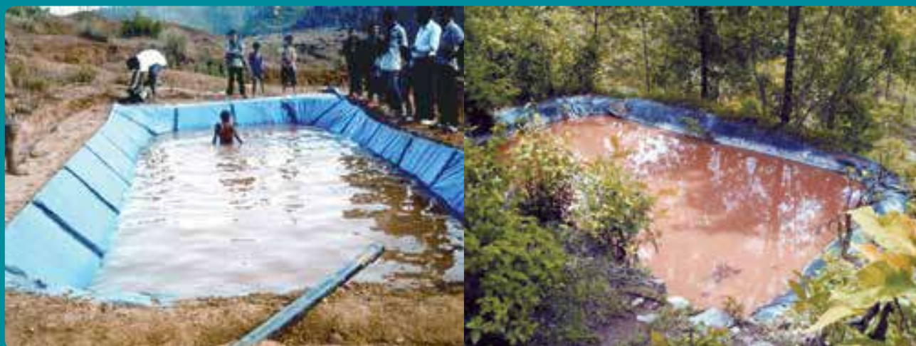
Figure 31: Earthen ponds laminated with plastic sheet
