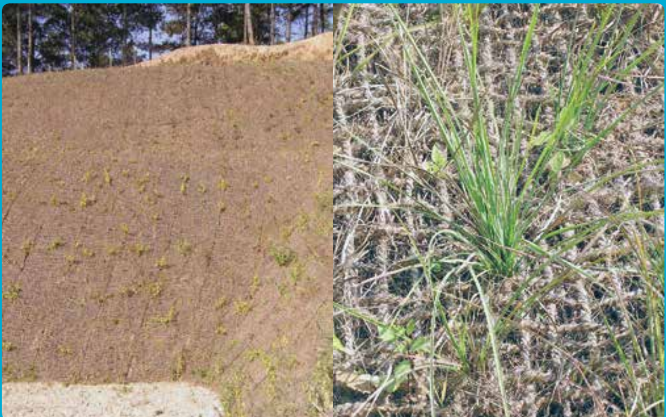
Figure 15: Jute netting on a cut slope
